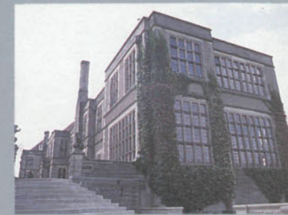
5. The main house from the north west.
