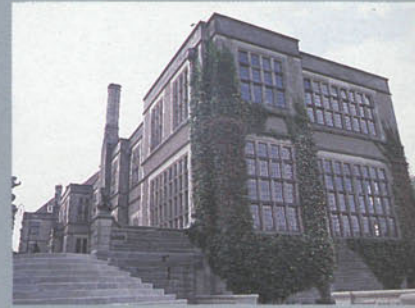
5. The main house from the north west.
