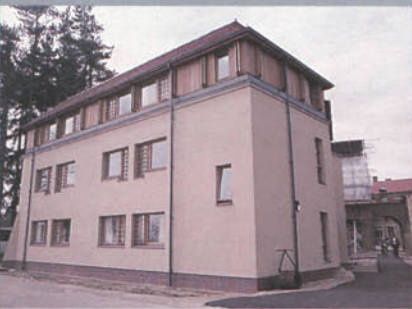
1. The new accommodation extension at the north east end of the annexe.
