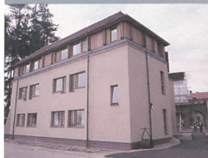
1. The new accommodation extension at the north east end of the annexe.
